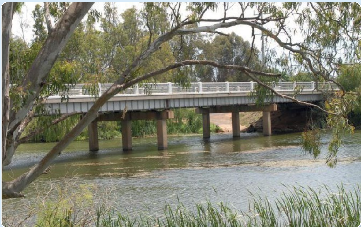
Bridgewater Bridge on Loddon
